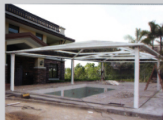
Build a framework
